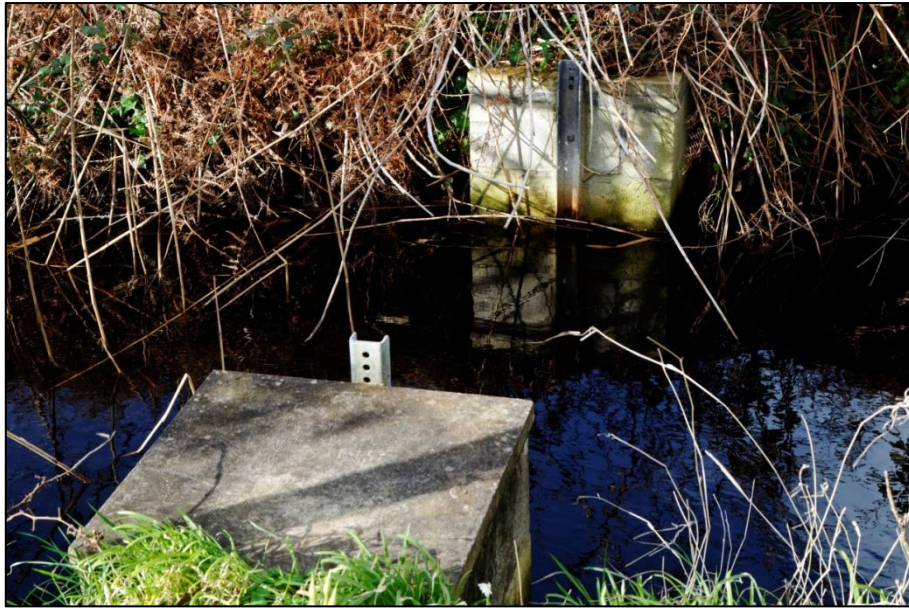
Figure 9 – Stop plank structure at the downstream point of the site boundary
